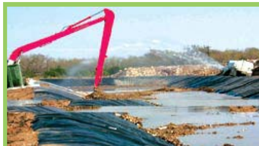
A pilot-scale study at the Naval Weapons Industrial Reserve Plant in McGregor, TX, evaluated ex situ treatment of perchlorate-contaminated soil and groundwater in a fixed-bed anaerobic bioreactor. ENSAFE, INC.
